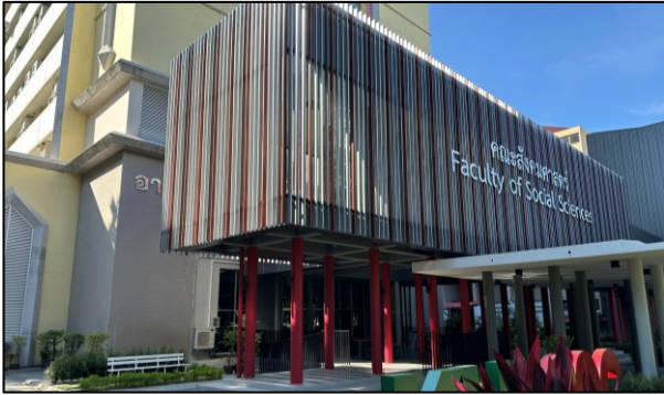
Fig 1. Photographs of the experimental building (Kasetsart University, Bangkok, Thailand, December 6, 2024).
